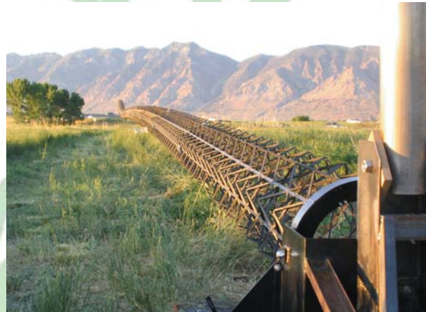
An IsoTruss tower, like this one waiting to go up, will be used by Dr. Tom Kolb for a flux tower. The towers are light, flexible and strong.
